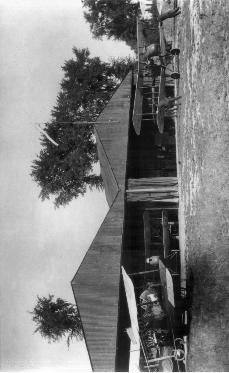
DH 2s of No 29 Sqn at Abeelee in 1916. The early aeroplanes were delicate, fragile and unreliable. Their integrity deteriorated rapidly when exposed to the elements, thus hangarage was essential.
