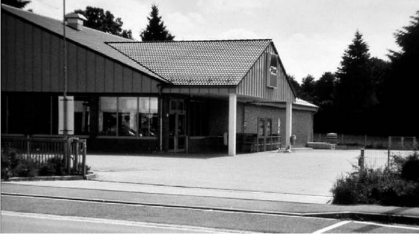
Above and opposite – a small supermarket and a straight stretch of road such as these constituted a viable WARLOC site.
