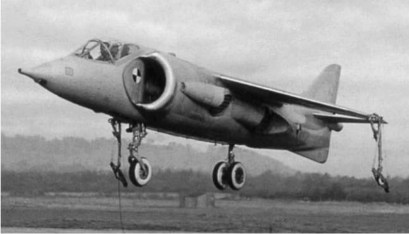
The first P1127, XP831, making an early tethered hover in 1960.
