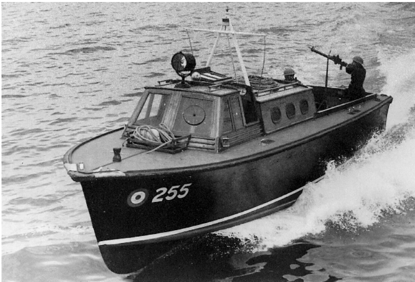
A 200 Class Seaplane Tender armed with a single Lewis gun. Aircraftman Shaw handled the trials of the lead boat in this class at Mount Batten. (Donald Smith)
