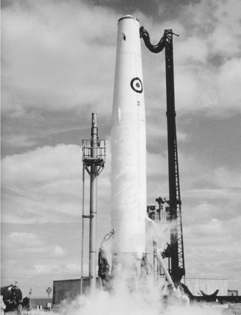
*LOX boiling off from one of No 113 Sqn's three Mepal-based missiles at T-4. Under peacetime conditions, only the oxidant was actually loaded during practice countdowns; the RP-1 fuel was also pumped but it by-passed the missile and was diverted into a tanker.*
