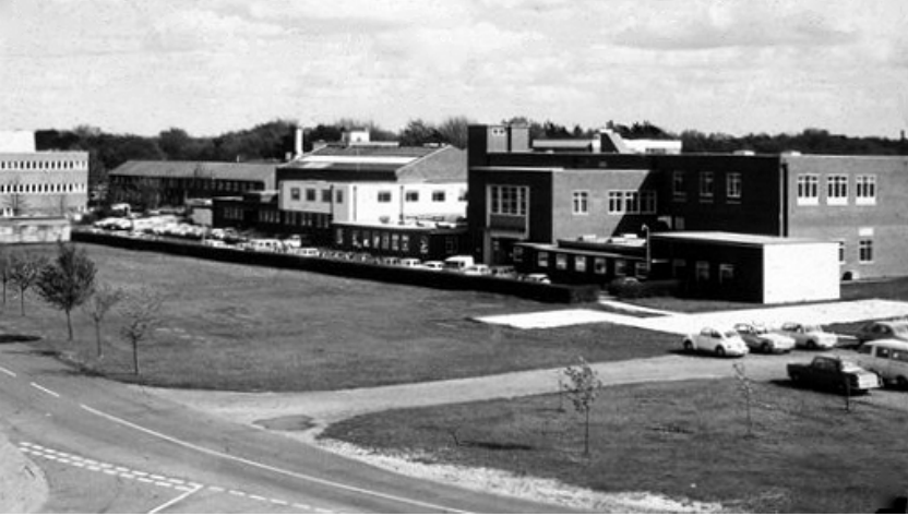
The old IAM complex at Farnborough which is being/has been demolished to make way for new development.
