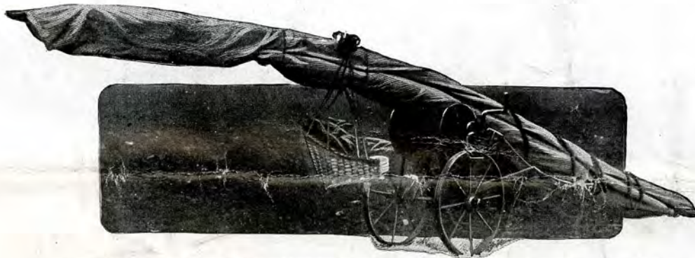
A complete outfit of man-lifting War Kites packed up ready for travel. They would be invaluable in time of war, as only eight men would be needed to draw them, and no carts or apparatus would be required as in ballooning.
