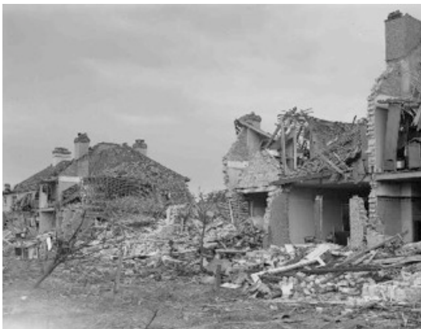
Result of a German flying bomb attack on a row of semi detached houses.
