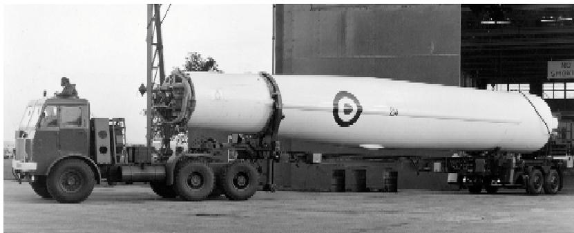
*Most Thor-associated equipment was trailer mounted, making the system 'portable', as distinct from 'mobile', not least because the launch emplacements themselves were very substantial fixed structures.*
