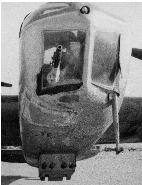
The field modification that provided the 20 mm cannon which was supposed to give the Blenheim IVF a notional anti-tank capability. It didn't. Note the four .303" Brownings in the belly pack.
