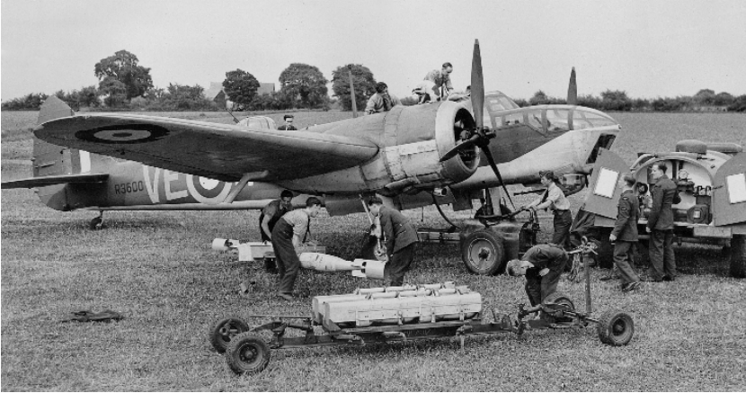
A long-nosed Blenheim IV of No 110 Sqn being loaded with 250 lb GP bombs and, in the foreground, a pair of Small Bomb Containers.
