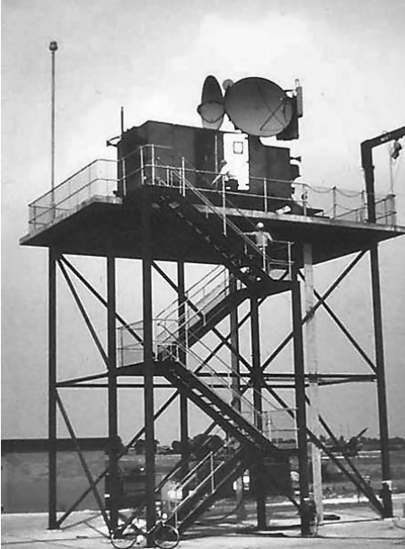
The Type 86 INDIGO CORKSCREW radar was vehicle mounted on a trailer to confer the degree of mobility required to support the Army's Thunderbird in the field. When used by the RAF at fixed sites, it was sometimes raised on a 30' platform, as here at Wattisham, to increase its low-level cover. (Nick Catford)
