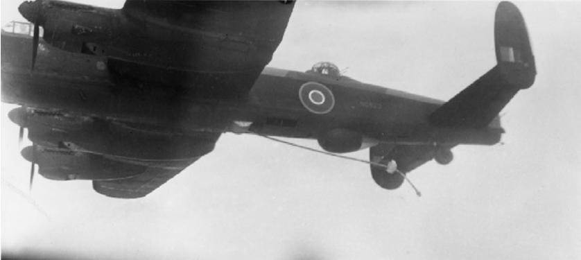
*Lancaster tanker seen from the receiver; the small drogue is to prevent the hose from whipping. Flight photo 18876s.*
