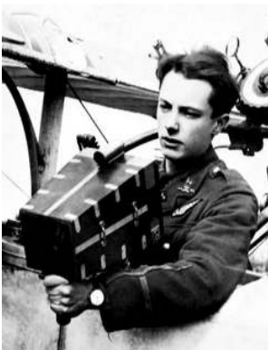
Left, the hand-held single-shot Type A camera; right, the magazine-fed Type C which was mounted on the airframe. (Barry Gray)
