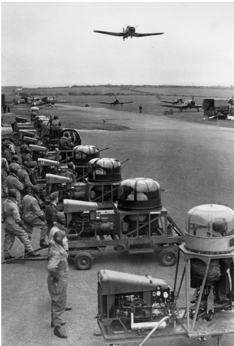
Turret training stands, a Bristol B1 at either end, but mostly Boulton Paul Type As plus at least one Type C (and, possibly, a Nash and Thompson FN64?), lined up at No 7 AGS, Stormy Down.
