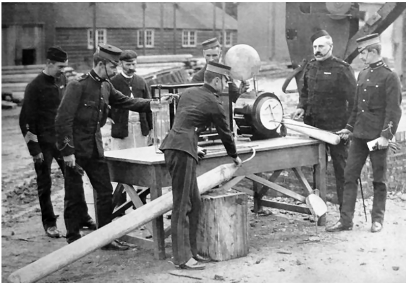
Lt Col Templer (second from right) overseeing the testing of a sample of hydrogen being drawn from a gas tube.
